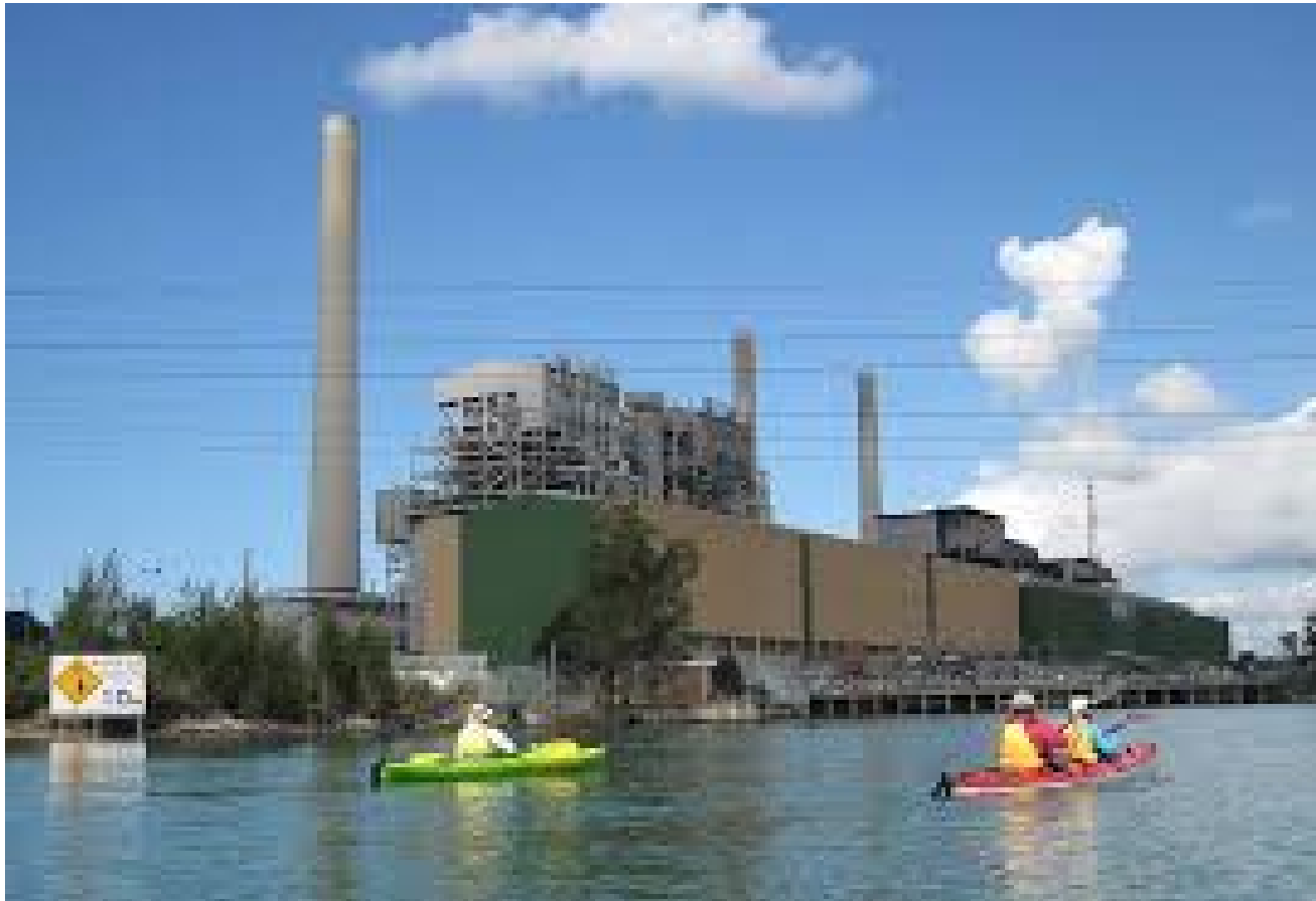
Coal Fired Generation – Vales Point (1320 MW = 2 x 660MW)
