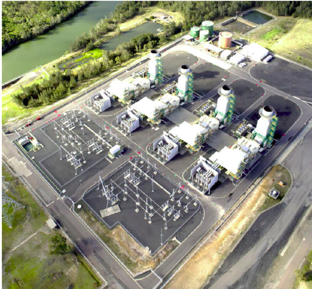
Open Cycle Gas Generation – Colongra (Munmorah region – 660MW = 4x165MW)
