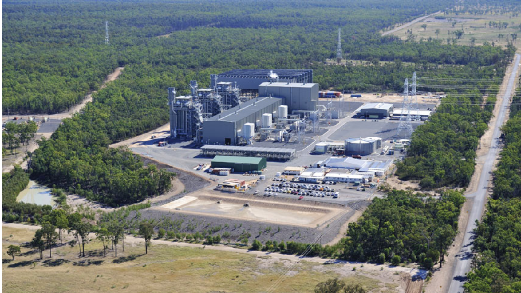
Combined Cycle Gas Generation – Darling Downs (630MW = 3x120MW+ 270MW)
