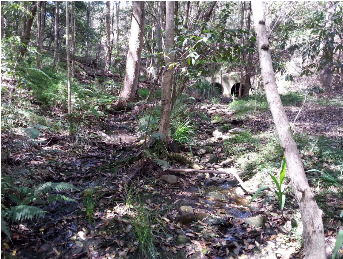
Inflow with drain pipes clearly visible
