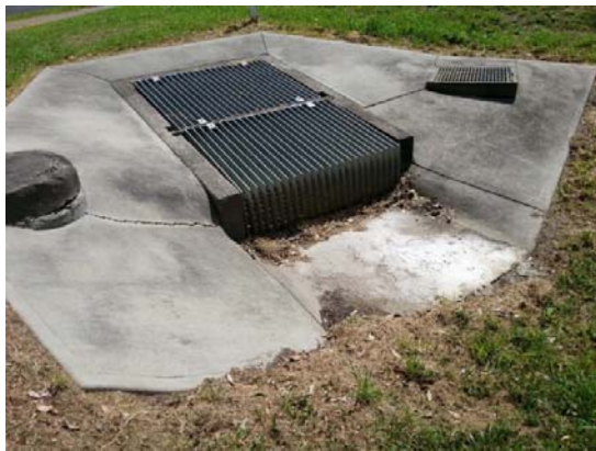
Sediment trap over drainage point
