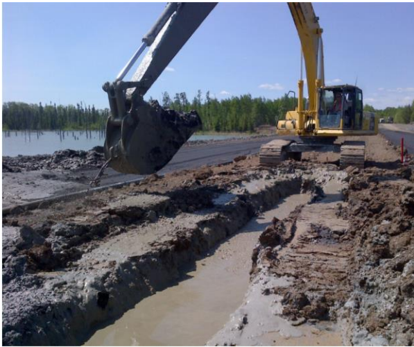
VALE Thompson Nickel Mine – Construction of the CB wall
