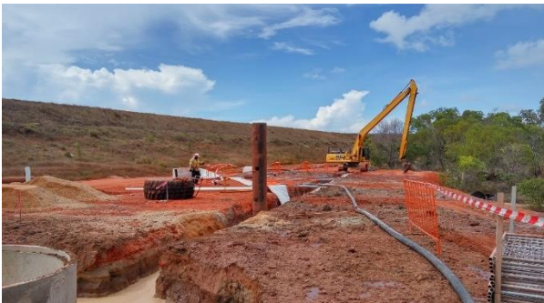
Rio Tinto – Construction of the SB wall
