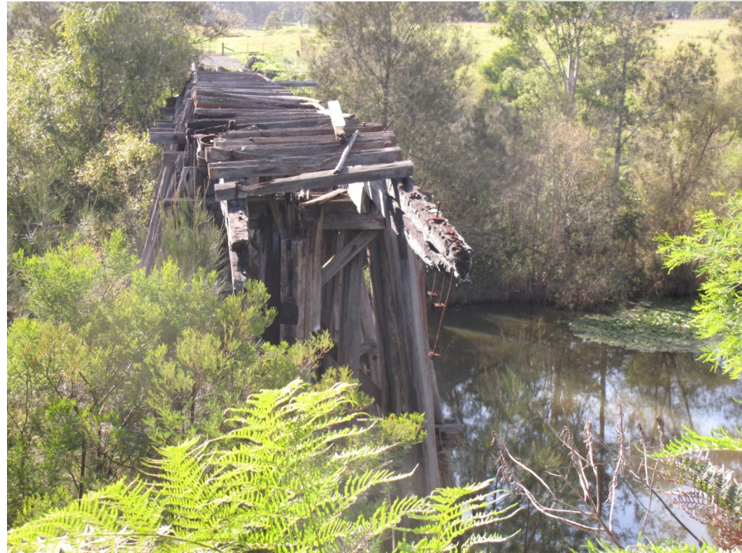
Avery's Bridge Wallis Creek
