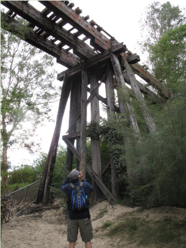
Burgess Bridge Surveyos Creek
